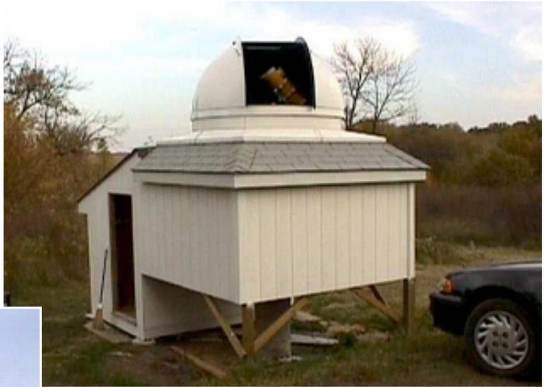
*Michael's astrograph can be seen through the opening in the dome. Access is through the door at ground level, then up to the observing floor. The concrete pedestal goes down far enough to reach stable ground somewhere near the Earth's mantle.*
